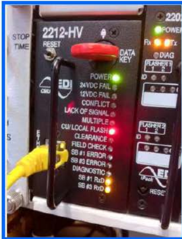
Output Assembly: CMU 2212-HV CU/LOCAL FLASH indicator is on
